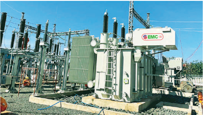
XÂY DỰNG TRẠM TRUYỀN TẢI 110KV/ Construction of transmission station 110kV
